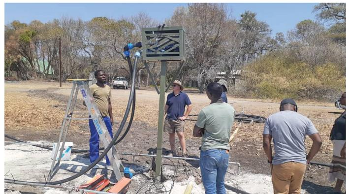
Installation of electric pumping system for shallow groundwater abstraction
