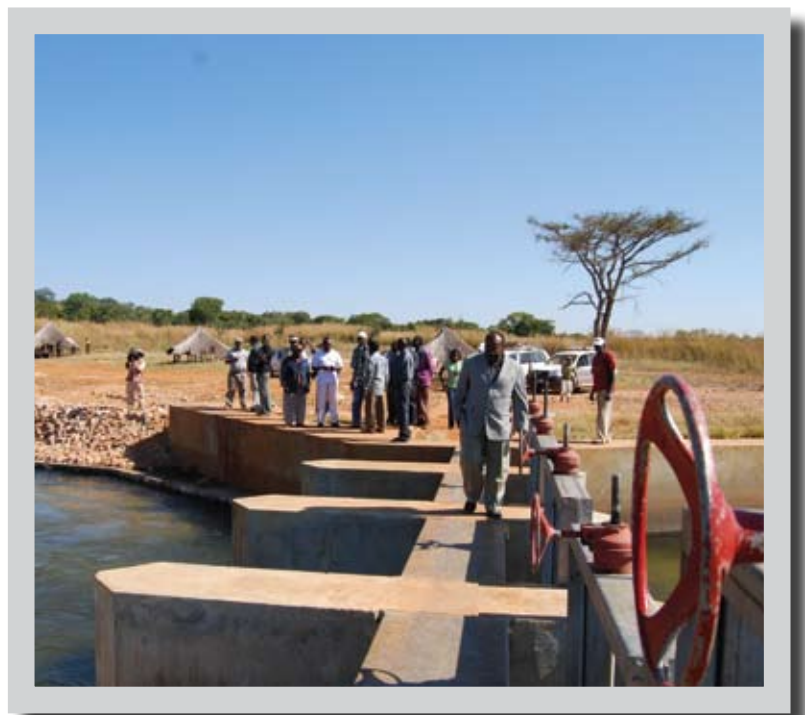
Water works at Menongue, Angola
